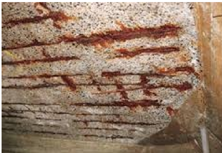
H 2 S corrosion taking a toll on the concrete walls, deteriorating the profile down to the rebar and potentially jeopardizing the integrity of the structure.
