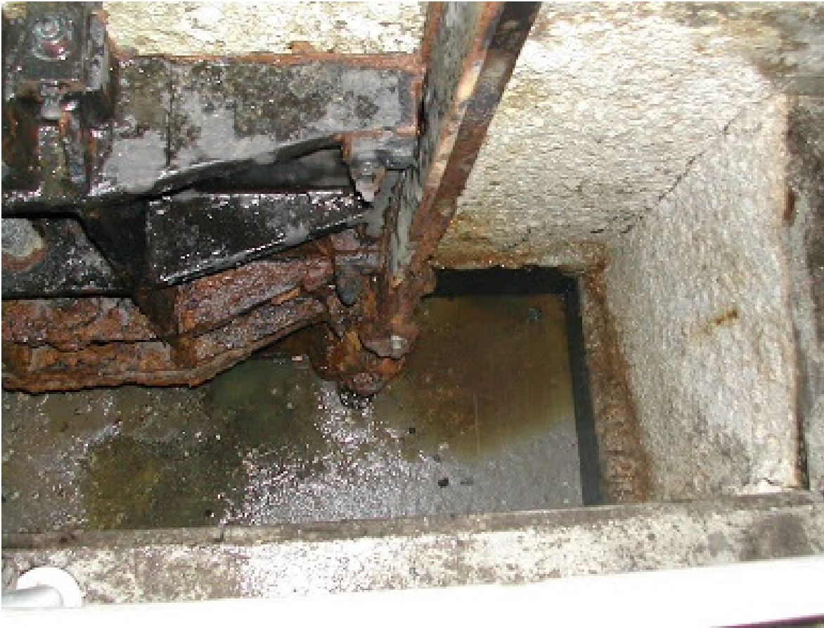
H 2 S corrosion taking a toll on the concrete walls, deteriorating the profile down to the rebar and potentially jeopardizing the integrity of the structure.
